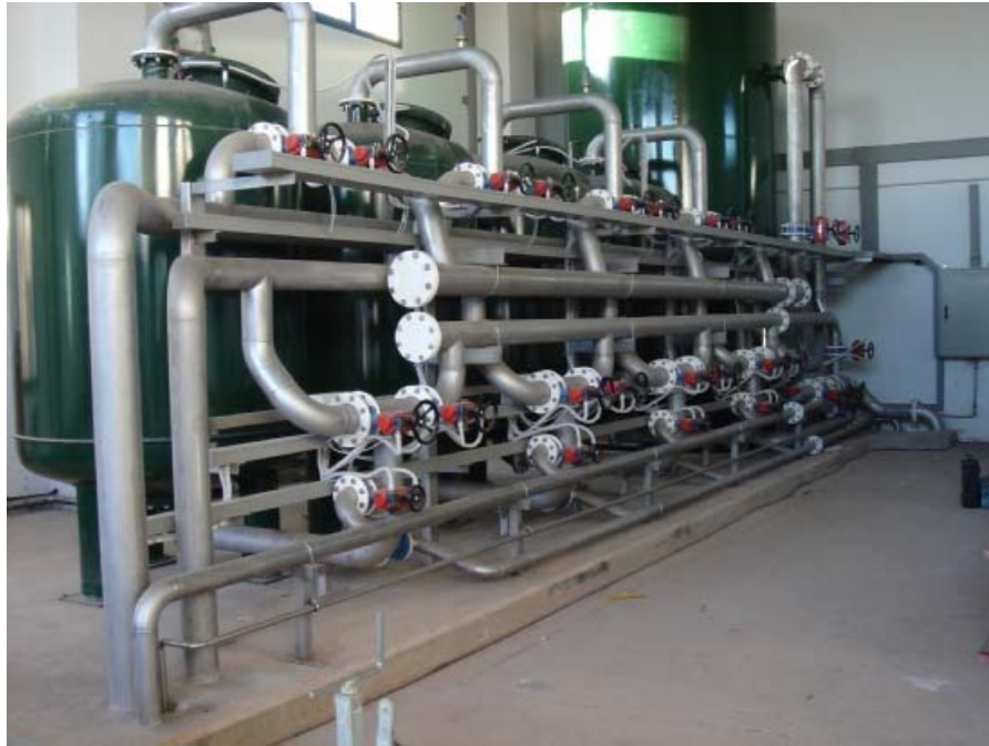
Figure 5. Overview of a pressure filter set. http://tecmoncade.com
